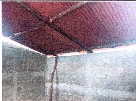
Foto 6: APROVECHAMOS LA CARA DEL MURO PERIMETRAL PARA CONTAR CON DICHA PARED
